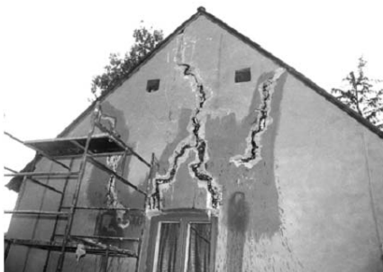
Figure 1. A detached house built in the area of intensive mining exploitation. Source: www.google.pl
