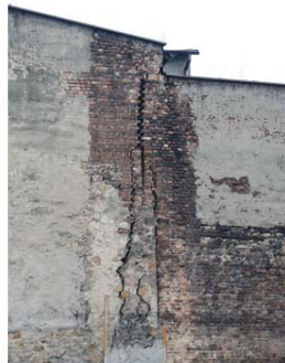
Figure 2. Multi-family house – a cracked supporting wall, in the area of intensive mining exploitation. Source: www.google.pl
