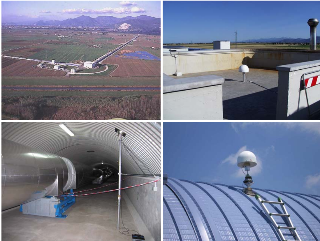
Fig. 6 – VIRGO master and GPS control points.
